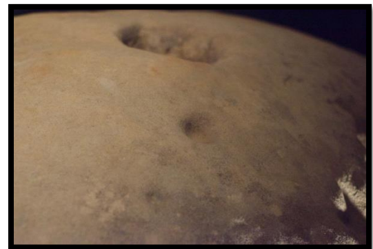
Photo 11: Nutting Hole with Larger Mortar Hole Behind
